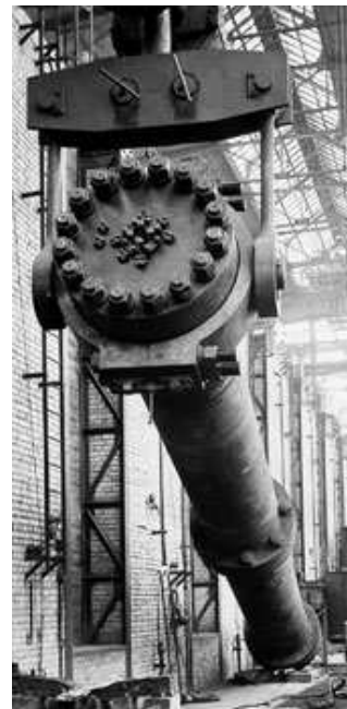
Installation of high-pressure reactor in the ammonia plant
